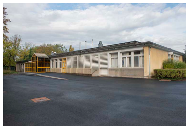
Angle sud-est de la restauration. Phot. Mary Ruffinoni IVR43_20139000019NUC4A
