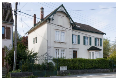
Logement patronal. Phot. Jérôme Mongreville IVR43_20122501837NUC4A
