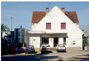
Pignon ouest. Phot. Jérôme Mongreville IVR43_19963900473ZA
