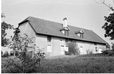
Logement patronal. Phot. Laurent Poupard IVR43_19883900569Z
