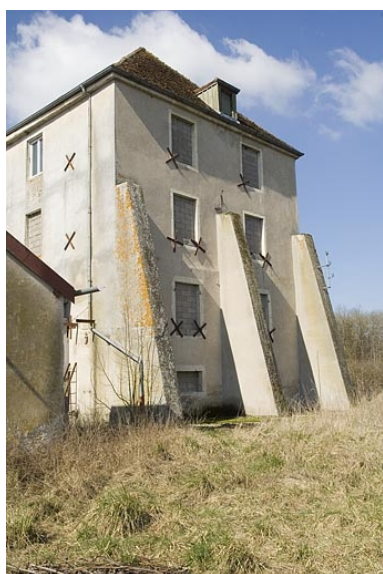
Contreforts sur le mur-pignon est. Phot. Jérôme Mongreville IVR43_20097000257NUC2A
