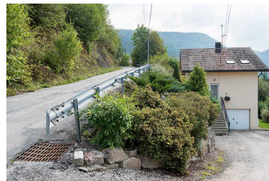
Façade nord. Phot. Sonia Dourlot IVR43_20162501279NUC4A
