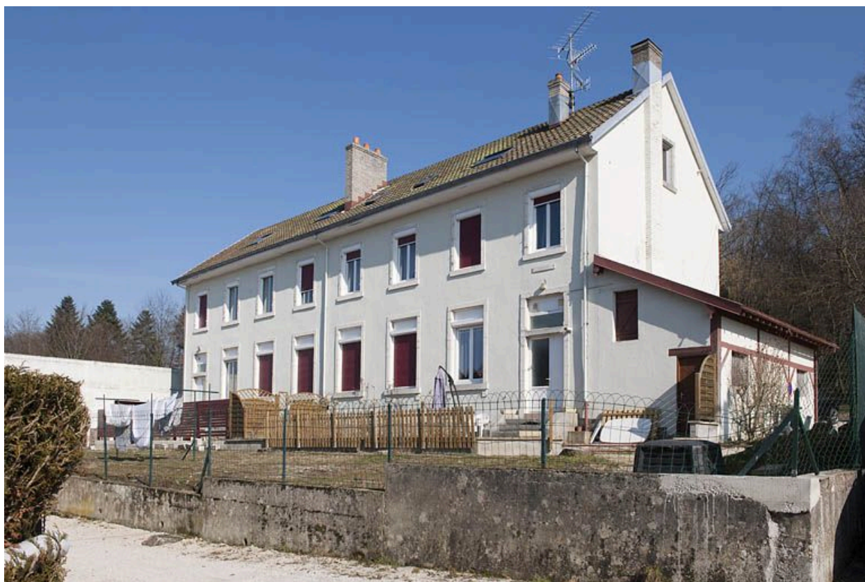
Ecole. Façade ouest.
