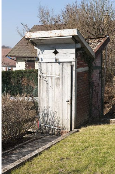
Latrines. Phot. Jérôme Mongreville IVR43_20122500152NUC4A
