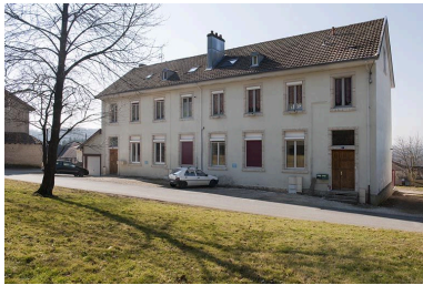
Ecole. Façade est. Phot. Jérôme Mongreville IVR43_20122500151NUC4A
