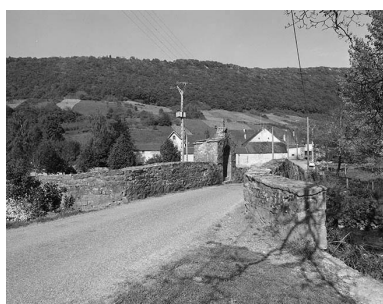
Tablier. Phot. Yves Sancey IVR43_19813900221X
