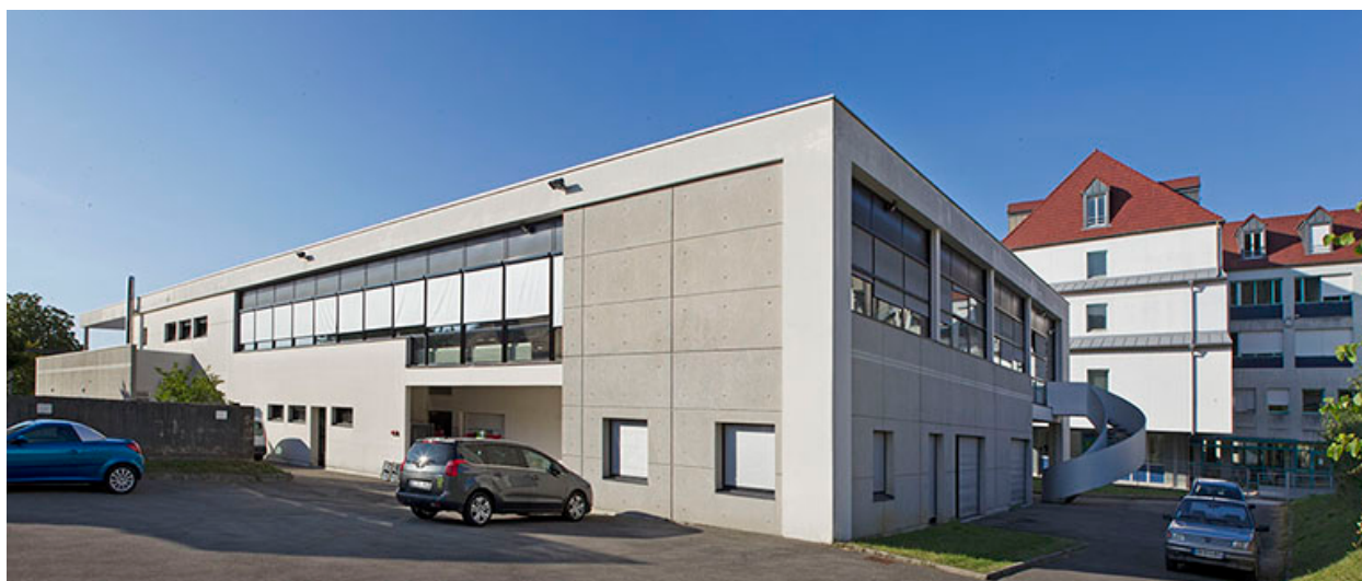
Restauration : façade Est.
