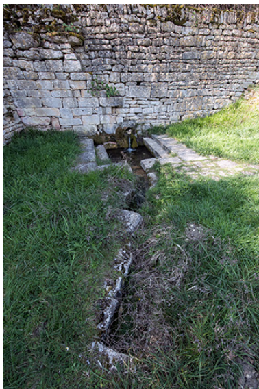
La fontaine de face. Phot. Nicolas Waltefaugle IVR26_20268900137NUC4A
