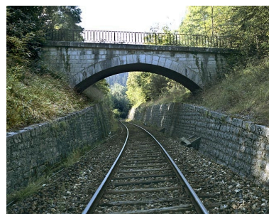
Elévation nord. Phot. Yves Sancey IVR43_20050100004XA
