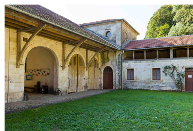
Revers du corps principal, angle sud. Phot. Sonia Dourlot IVR43_20167000767NUC2A
