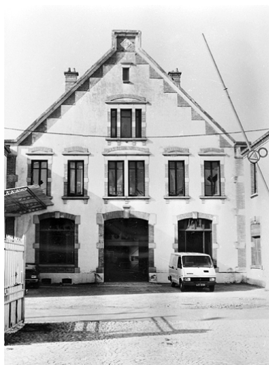
Ateliers sud-est. Phot. Jérôme Mongreville IVR43_20019000114X
