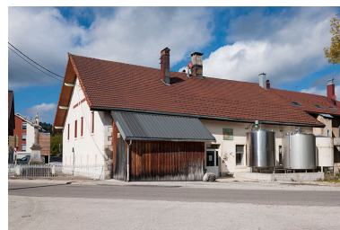
Façade est. Phot. Jérôme Mongreville IVR43_20152501893NUC4A
