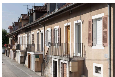
Elévation de la façade est. Phot. Jérôme Mongreville IVR43_20112502236NUC4A
