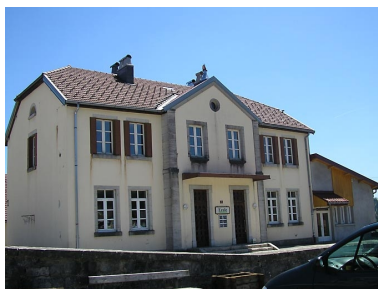
Mairie. Phot. Marie-Pierre Reynet IVR43_20083900292NUC1A
