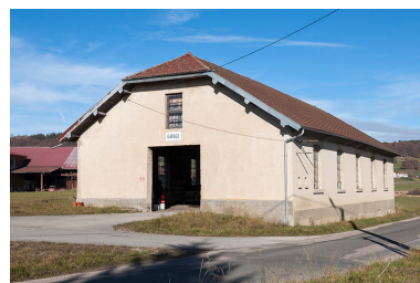
Garage. Phot. Jérôme Mongreville IVR43_20152502383NUC4A
