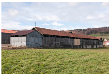
Hangars de stockage. Phot. Jérôme Mongreville IVR43_20152502403NUC4A
