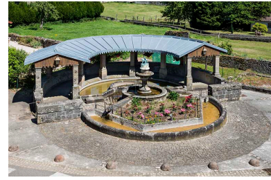
Fontaine-lavoir, Ferrières-lès-Scey. Phot. Jérôme Mongreville IVR43_20177000806NUC4A
