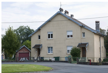
Logement double. Phot. Jérôme Mongreville IVR43_20122501849NUC4A
