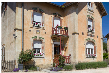
Façade antérieure. Phot. Sonia Dourlot IVR43_20157000313NUC2A
