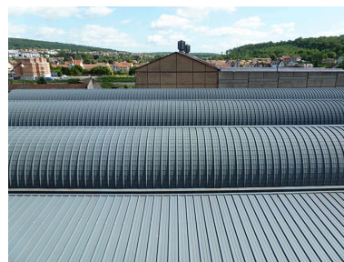
Toiture des ateliers. Phot. Mary Ruffinoni IVR43_20147000044NUC4A
