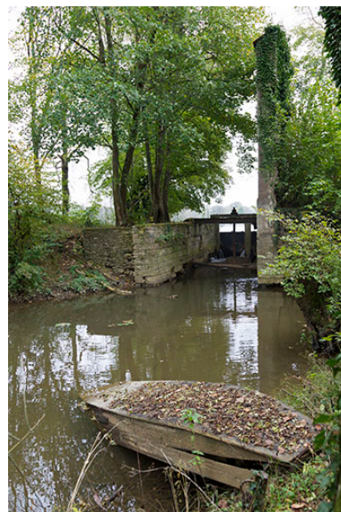
Ancien moulin. Phot. Sonia Dourlot IVR43_20157000127NUC2A
