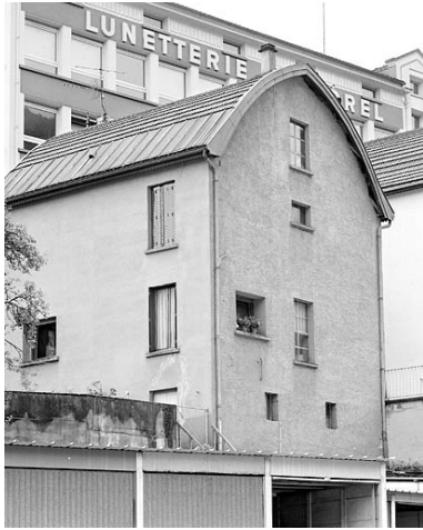
Façade postérieure. Phot. Yves Sancey IVR43_20033900204X
