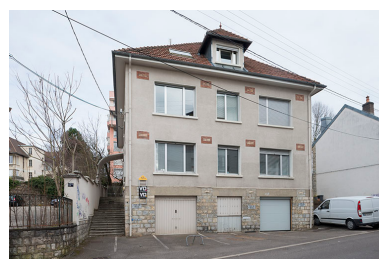
Façade est. Phot. Jérôme Mongreville IVR43_20182500529NUC4A
