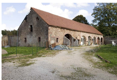
Ecuries et remises. Phot. Jérôme Mongreville IVR43_20077000515NUCA
