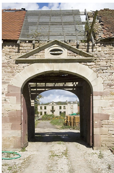
Portail. Phot. Jérôme Mongreville IVR43_20077000510NUCA
