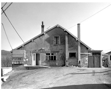
Façade sud. Phot. Yves Sancey IVR43_19973900558X
