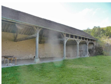
Hangar. Phot. Cécile Lestienne, Phot. Virginie Malherbe IVR26_20128900289NUC2A
