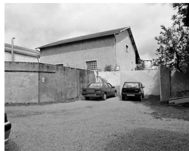
Entrepôt industriel. Phot. Yves Sancey IVR43_20009000068X
