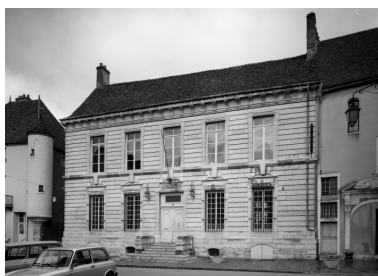
Façade. Phot. Michel Rosso IVR26_19862100093V
