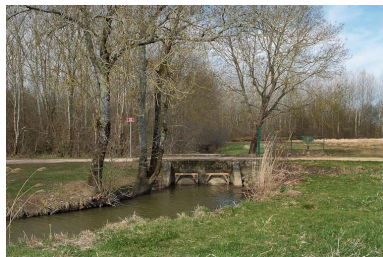
Le pont. Phot. Jean-Luc Duthu IVR26_20107100389NUC2A
