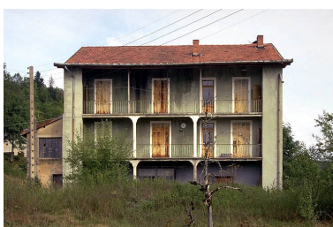
Logement. Phot. Laurent Poupard IVR43_19913901281ZA
