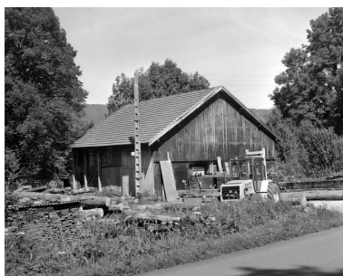
Magasin industriel. Phot. Yves Sancey IVR43_19973901233X
