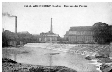
12348. AUDINCOURT (Doubs) - Barrage des Forges. Carte postale. Phot. Yves Sancey IVR43_19842500144X
