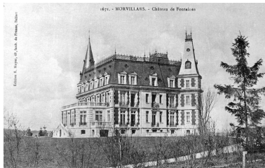
Morvillars. Château de Fontaines. Phot. Jérôme Mongreville IVR43_20019000105X
