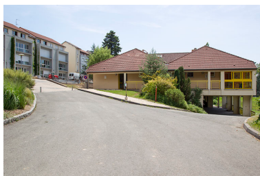
Façade nord de la restauration. Phot. Jérôme Mongreville IVR43_20149000193NUC2A
