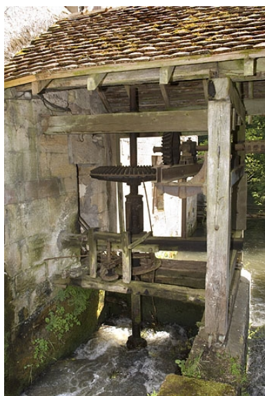
Local de la turbine. Phot. Jérôme Mongreville IVR43_20097000647NUC2A
