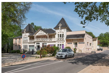
façade principale. Phot. Pierre-Marie Barbe-Richaud IVR26_20222100206NUC4A
