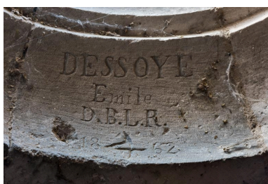
Comble, graffiti : Dessoye Emile D.B.L.R. 1862. Phot. Pierre-Marie Barbe-Richaud IVR26_20222100452NUC4A
