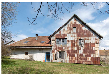
Façade ouest. Phot. Sonia Dourlot IVR43_20192500326NUC4A
