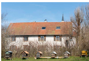
Façade sud. Phot. Sonia Dourlot IVR43_20192500328NUC4A
