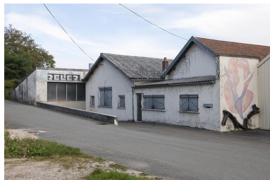
Ateliers de fabrication. Phot. Jérôme Mongreville IVR43_20122501834NUC4A
