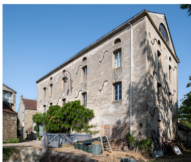
Le pignon oriental. Phot. Nicolas Waltefaugle IVR26_20268900371NUC4A
