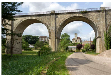
Le viaduc. Phot. Sonia Dourlot IVR43_20157000581NUC2A
