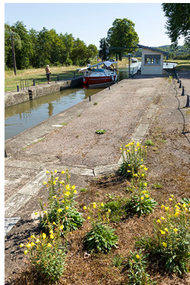
L'écluse. Phot. Sonia Dourlot IVR43_20157000729NUC2A
