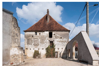
Mur pignon sud. Phot. Jérôme Mongreville IVR43_20167000443NUC4A
