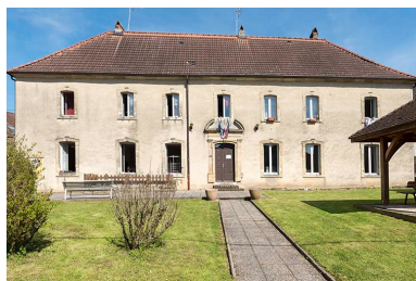
Façade principale. Phot. Sonia Dourlot IVR43_20167000553NUC4A
