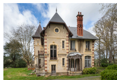
Façade est. Phot. Pierre-Marie Barbe-Richaud IVR26_20245800176NUC4A
