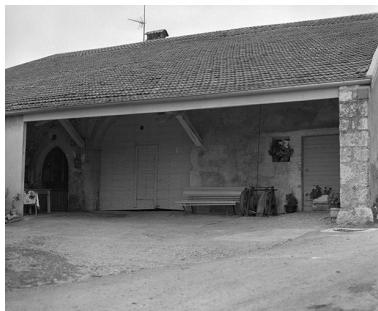
Mur goutterot. Phot. Yves Sancey IVR43_19782500396X
