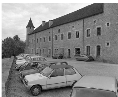
Façade ouest. Phot. Yves Sancey IVR43_19813900088X
