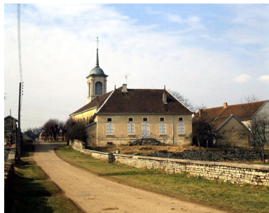
Façade postérieure. Phot. Yves Sancey IVR43_19857000100XA
