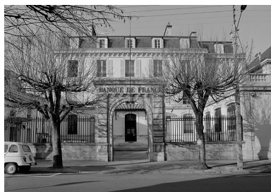
La Banque de France. Phot. Yves Sancey IVR43_19833900621X
